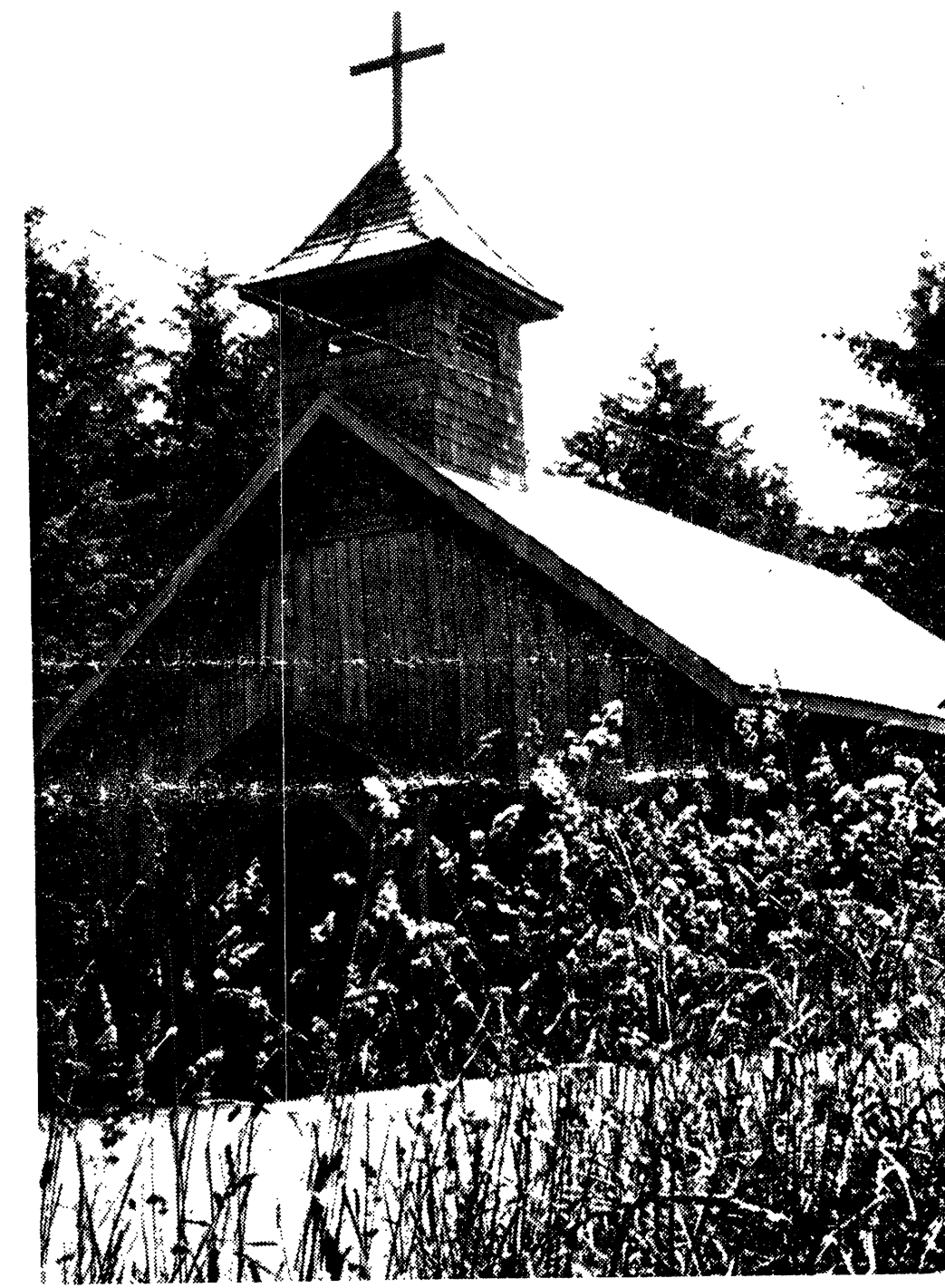
CONDEMNED--This old Shaker Church built in 1917 served LaPush for more than 45 years both as a house of worship and a community hall. Lumber for this structure was purchased at Iversons Mill near Forks with contributions by Jim Ward and many people of the Quillayute Reservation. Lumber was taken by horse team from the mill at Mill Creek to the Bogachiel River then by canoe on to LaPush. Hal George who at that time was manager of the Quillayute Braves baseball team, still recalls the long journey down river and the many hours spent with his hall team constructing their new church. Standing somewhat unstable, this old landmark will someday crumble under the powerful Pacific winds. by Lonnie Archibald
